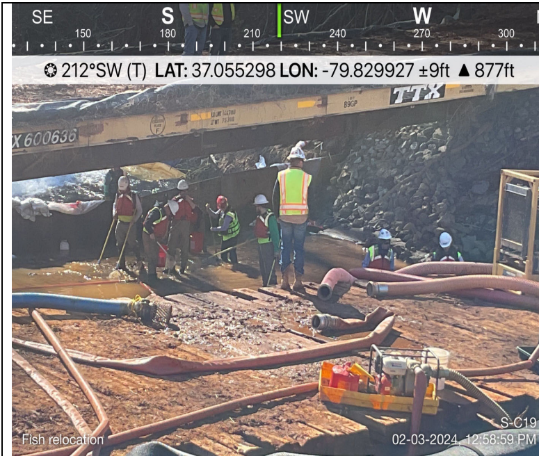
Photo Description: Fish relocation crew on-site removing fish after construction area isolated with dam & pump.
