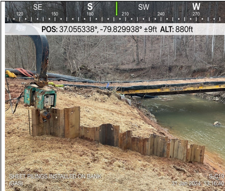
Photo Description: Sheet pilings (GAS).
