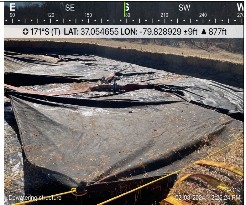
Photo Description: Dewatering structure installed and utilized on-site throughout pipe installation.
