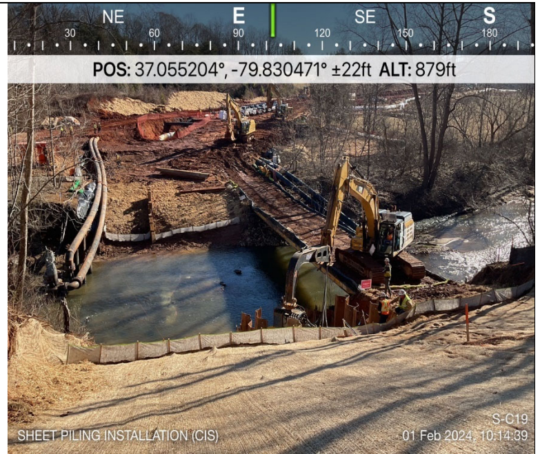
Photo Description: Installation of sheet piles (CIS).
