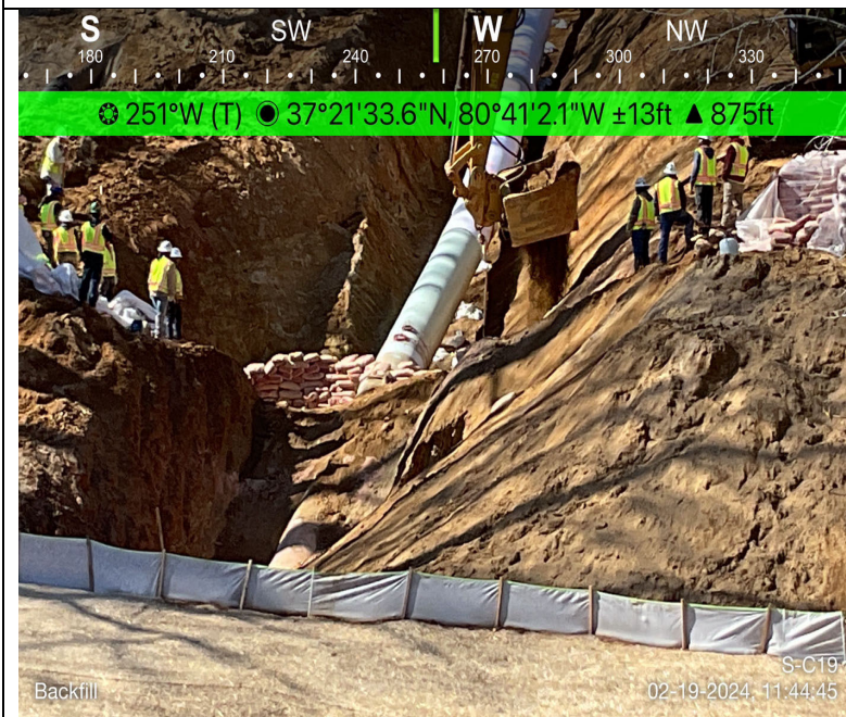
Photo Description: Backfill CIS of resource crossing.
