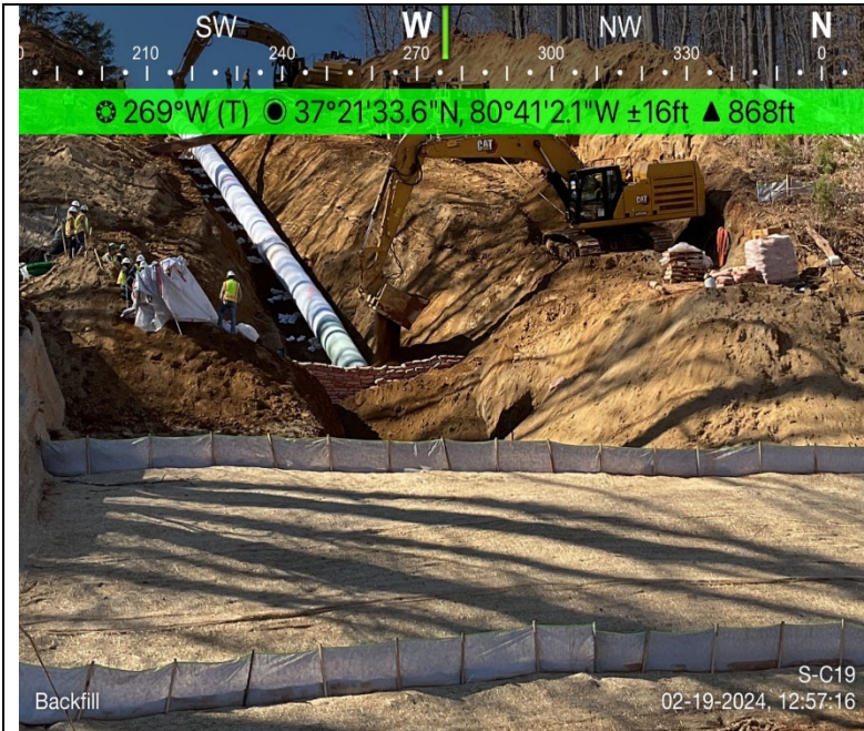
Photo Description: Trench breaker installation on CIS
