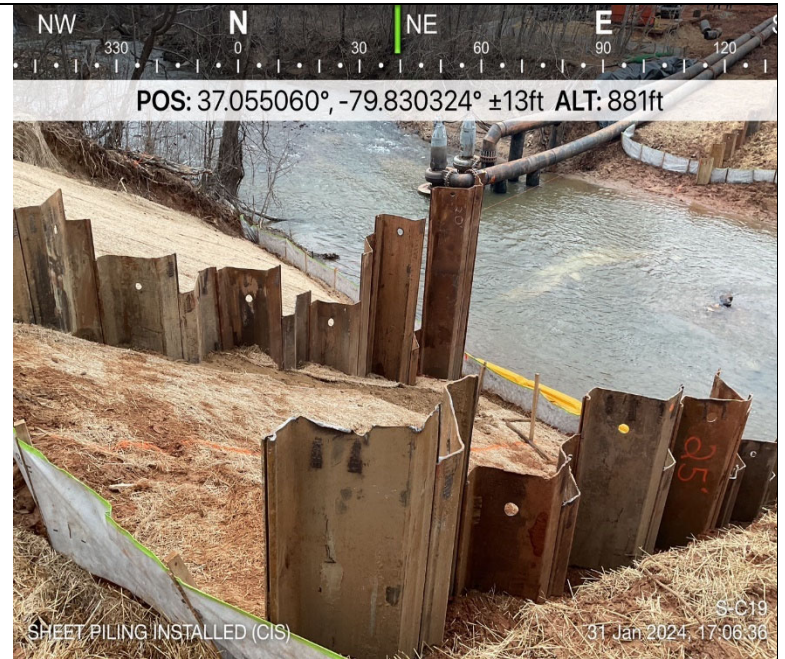
Photo Description: Sheet pilings (CIS).
