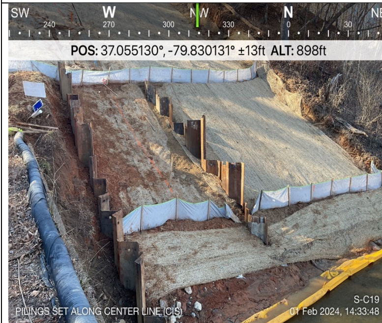
Photo Description: Installation of sheet piles (CIS).
