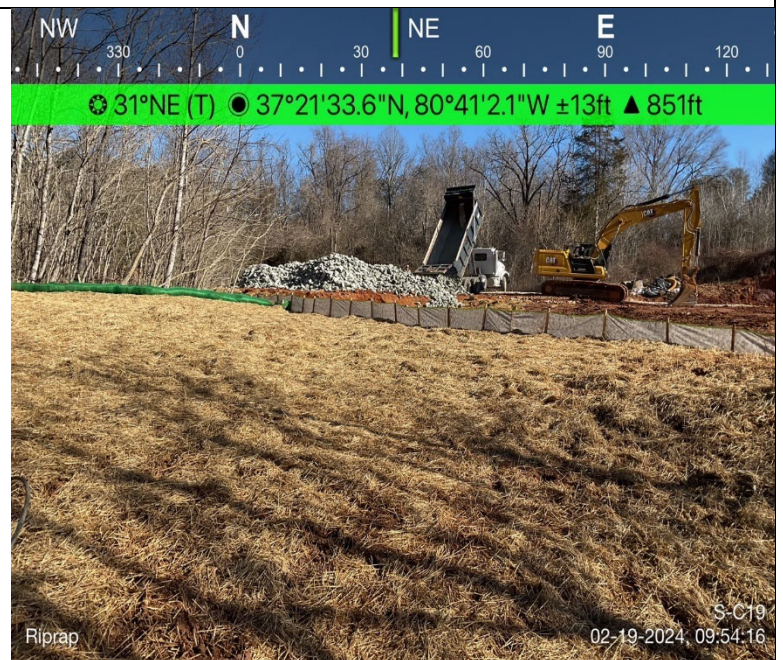
Photo Description: Riprap for stream banks staging on-site.
