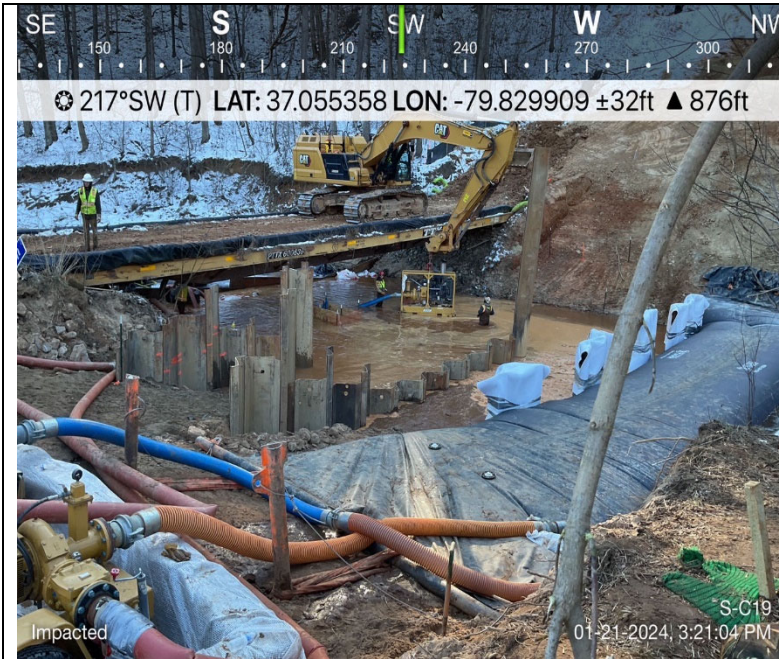
Photo Description: Stream overflowed downstream dam.
