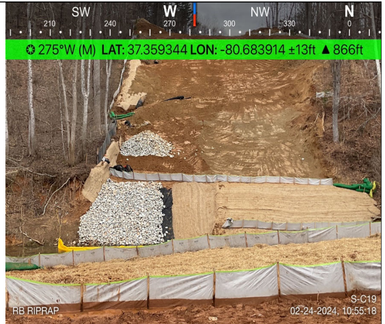
Photo Description: Riprap installation underway on right bank of resource.
