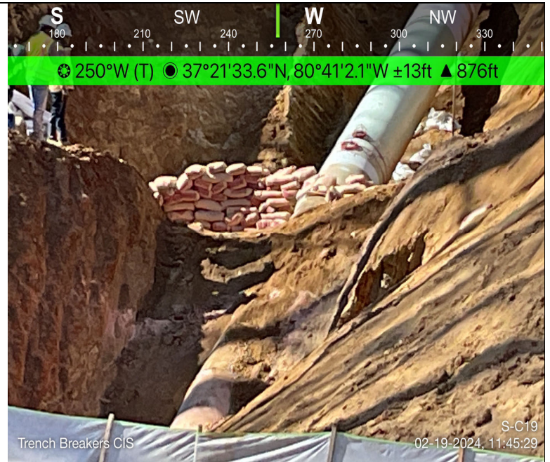
Photo Description: Trench breakers installation on CIS.
