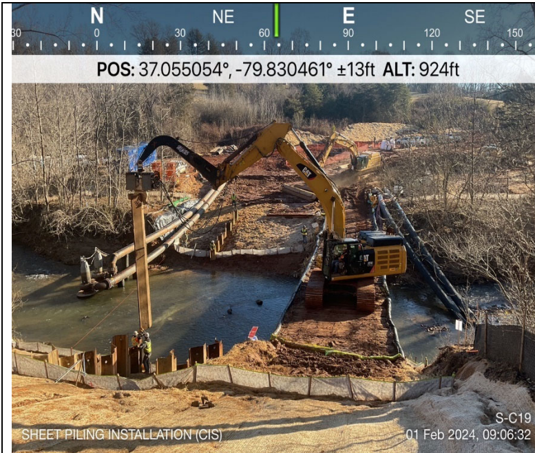
Photo Description: Installation of sheet piles (CIS).
