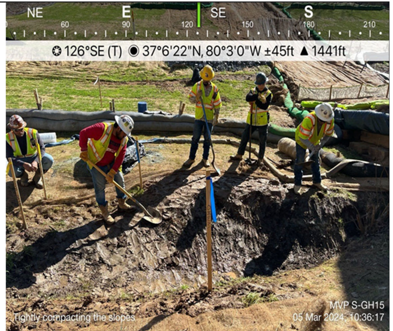
Photo Description: Both banks were graded to a more gradual slope and compacted.
