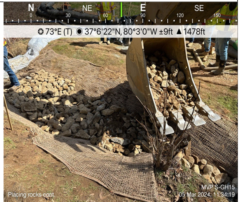
Photo Description: Native stream bed rock from S-D11 crossing was placed in the stream bed to enhance stabilization.
