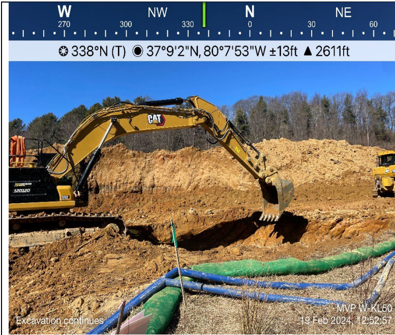
Photo Description: The topsoil was excavated.
