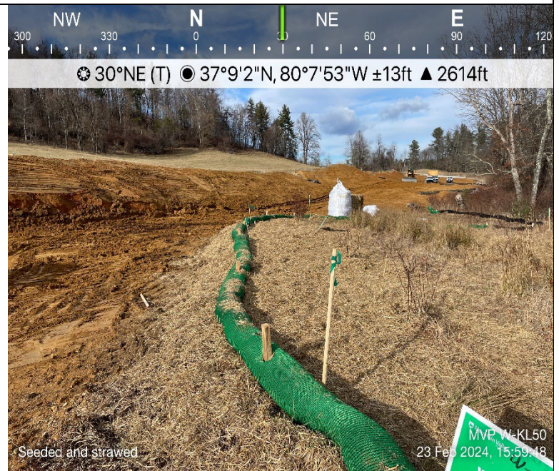
Photo Description: The area was restored with seed, straw mulch, and compost filter sock.
