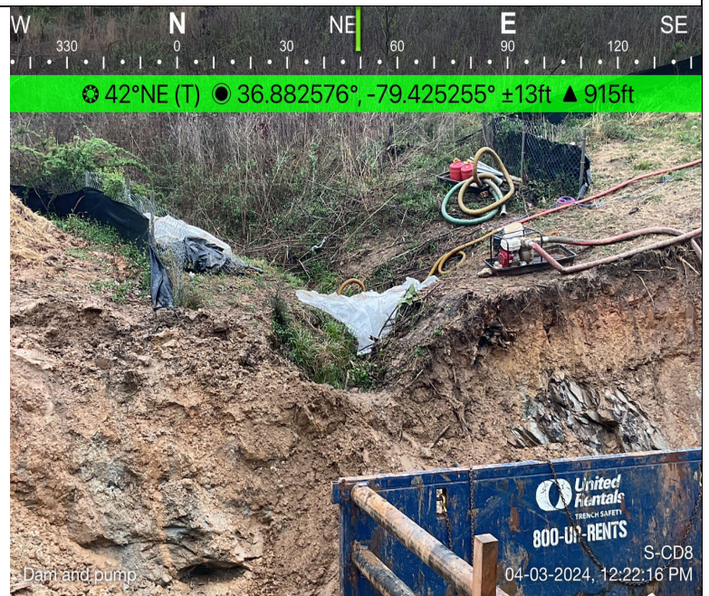
Photo Description: An overview of the dam and pump.
