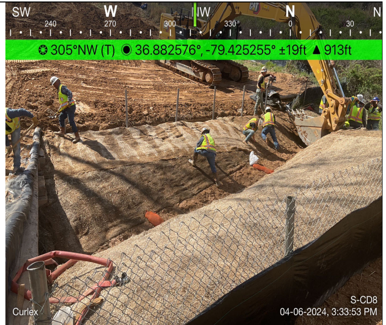
Photo Description: Curlex matting was installed along the stream bank.
