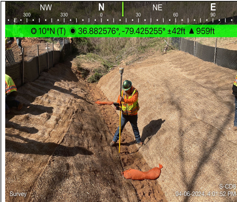
Photo Description: Survey of the substrate post-construction.
