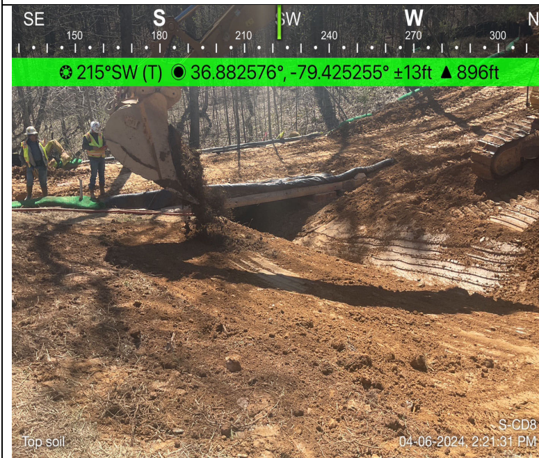
Photo Description: Topsoil was returned to the stream bank and graded.
