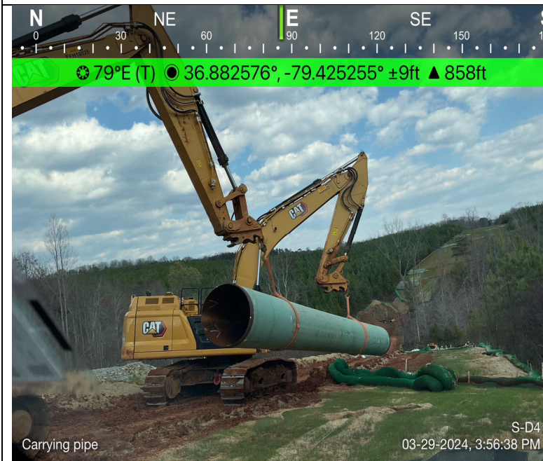
Photo Description: Pipe being transported to the trench for anomaly replacement.
