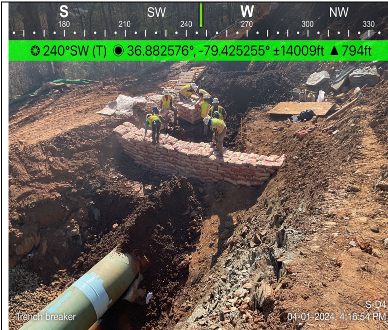
Photo Description: The trench breaker was installed along the pipe.
