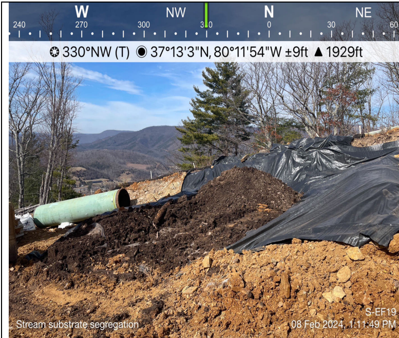
Photo Description: Stream substrate segregation and stockpiled on fabric in upland area.
