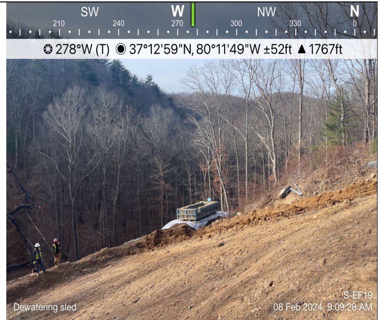
Photo Description: Dewatering sled on-site throughout the crossing activities.
