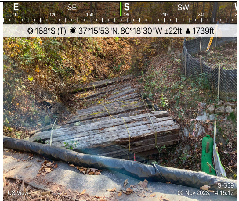
Photo Description: Upstream view with old deck mats to be removed.
