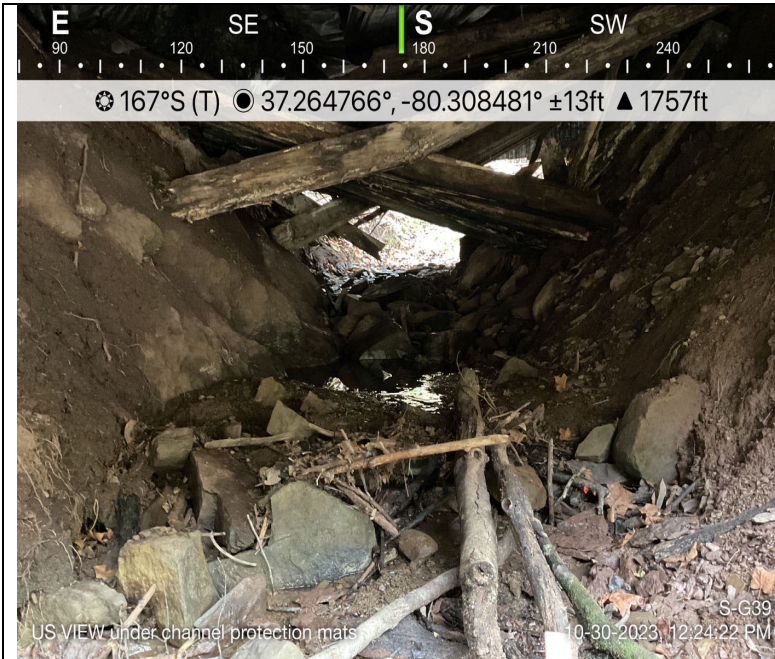
Photo Description: Upstream view under channel protection mats.
