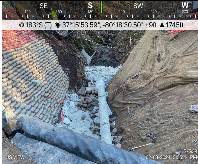
Photo Description: Upstream view of the resource impact area from the timber mat bridge. Highwall installation continues while resource is flumed and plastic in resource to catch debris from upslope.
