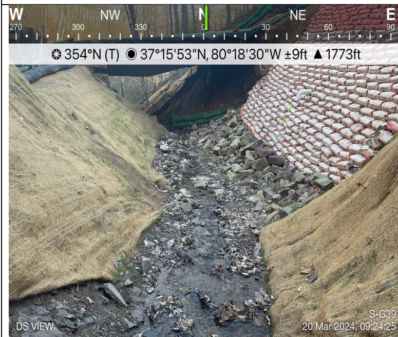
Photo Description: Downstream view of permitted impact area during post-construction assessment.
