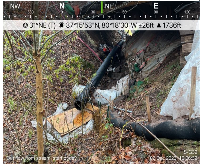
Photo Description: Flume outfall onto non-erodible material to prevent downstream scour.
