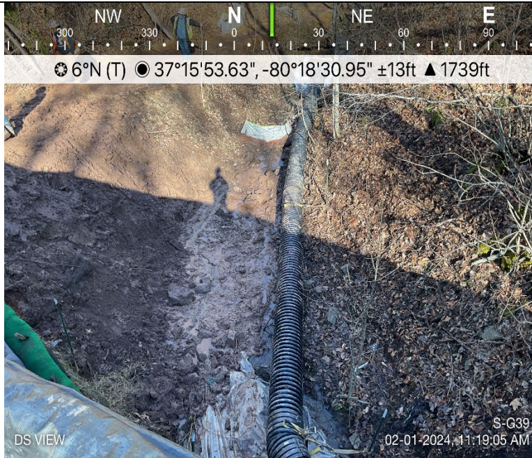
Photo Description: Material from right of way slip was retrieved down to the original stream substrate.
