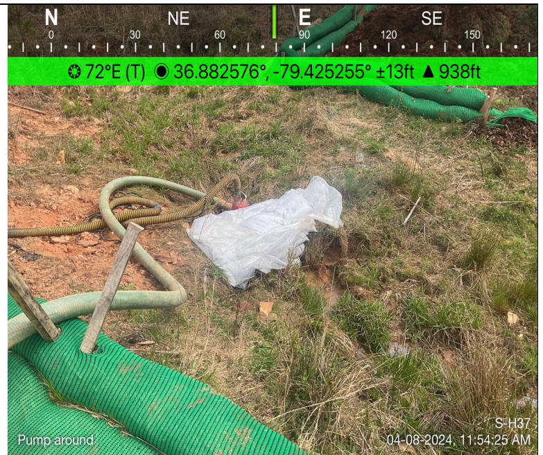
Photo Description: Dam and pump installed prior to resource disturbance.
