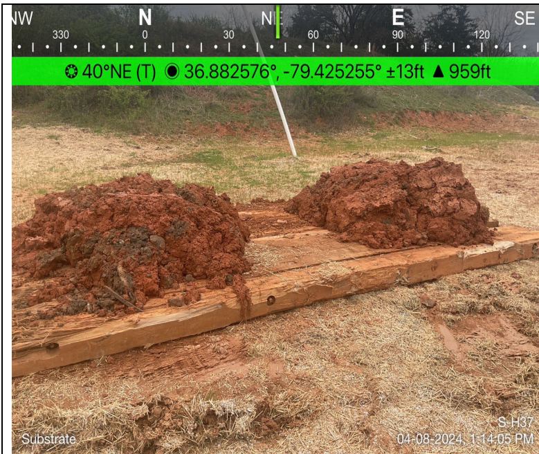
Photo Description: Substrate segregation from other soils during work activities.
