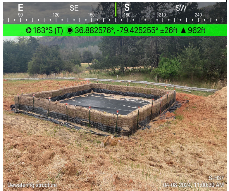
Photo Description: Dewatering structure installed on-site.
