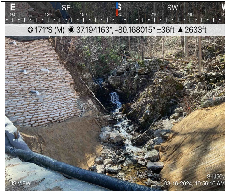
Photo Description: Upstream view of permitted impact area during post-construction assessment.
