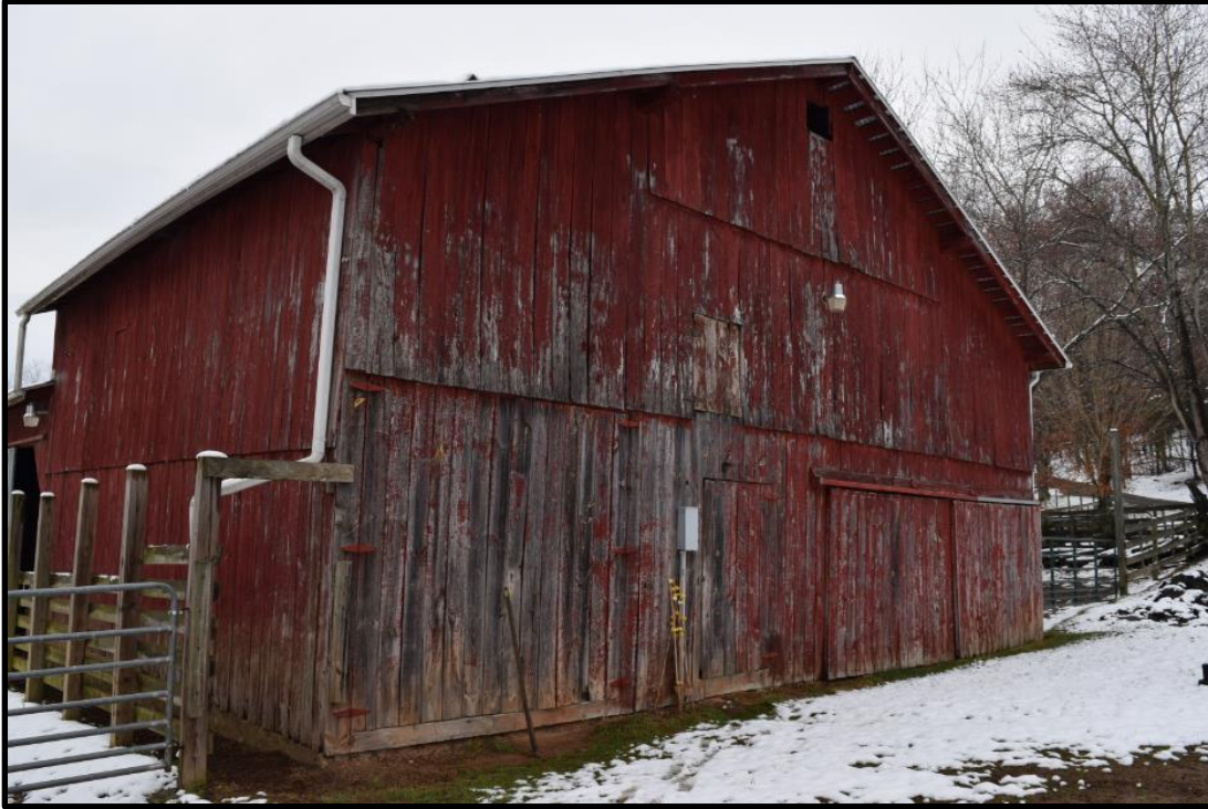
Figure 4: Barn at 3157 Booker T. Washington Highway (Route 122) Rocky Mount, Franklin County, View Southeast
